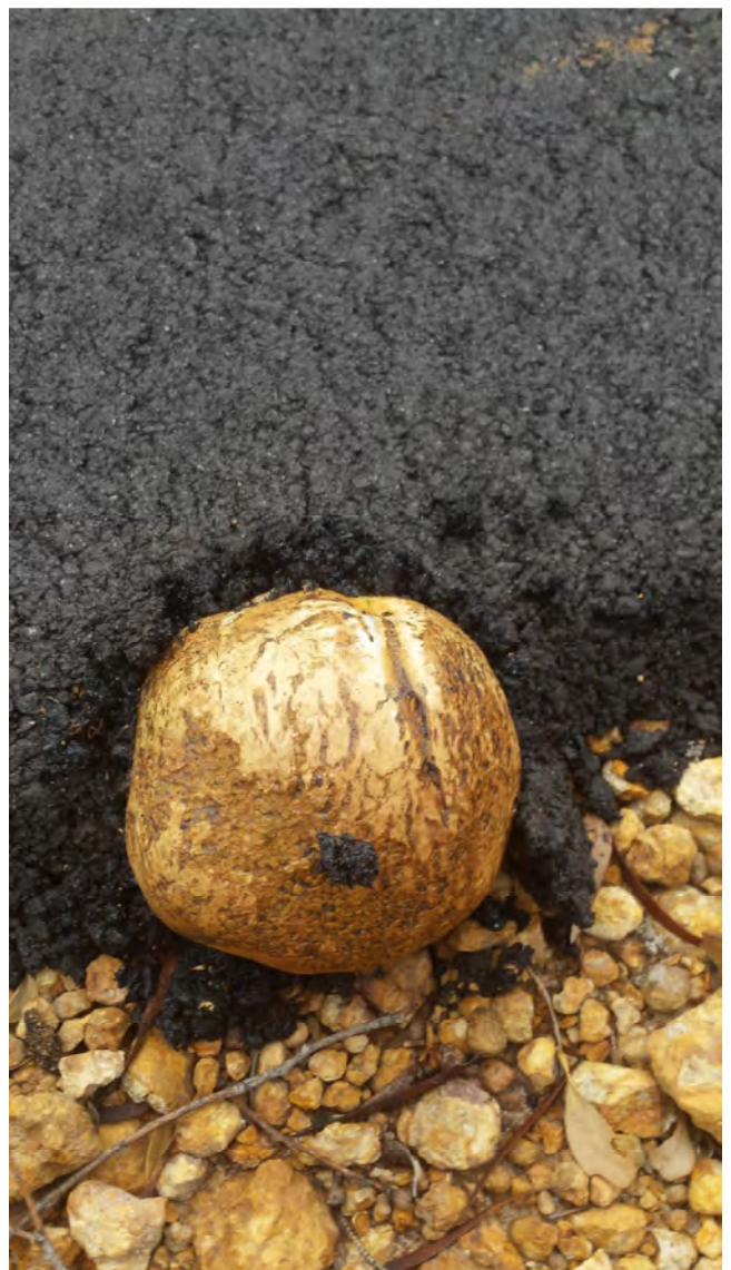
Pisolithus breaking through the new bitumen bike track in Bremer Bay (Images: J. Messina).
